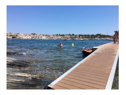
The Unideck ® system consists of structures made of aluminum, corrosion resistant, covered with decking and optionally bonded together by silent armed blocks.
